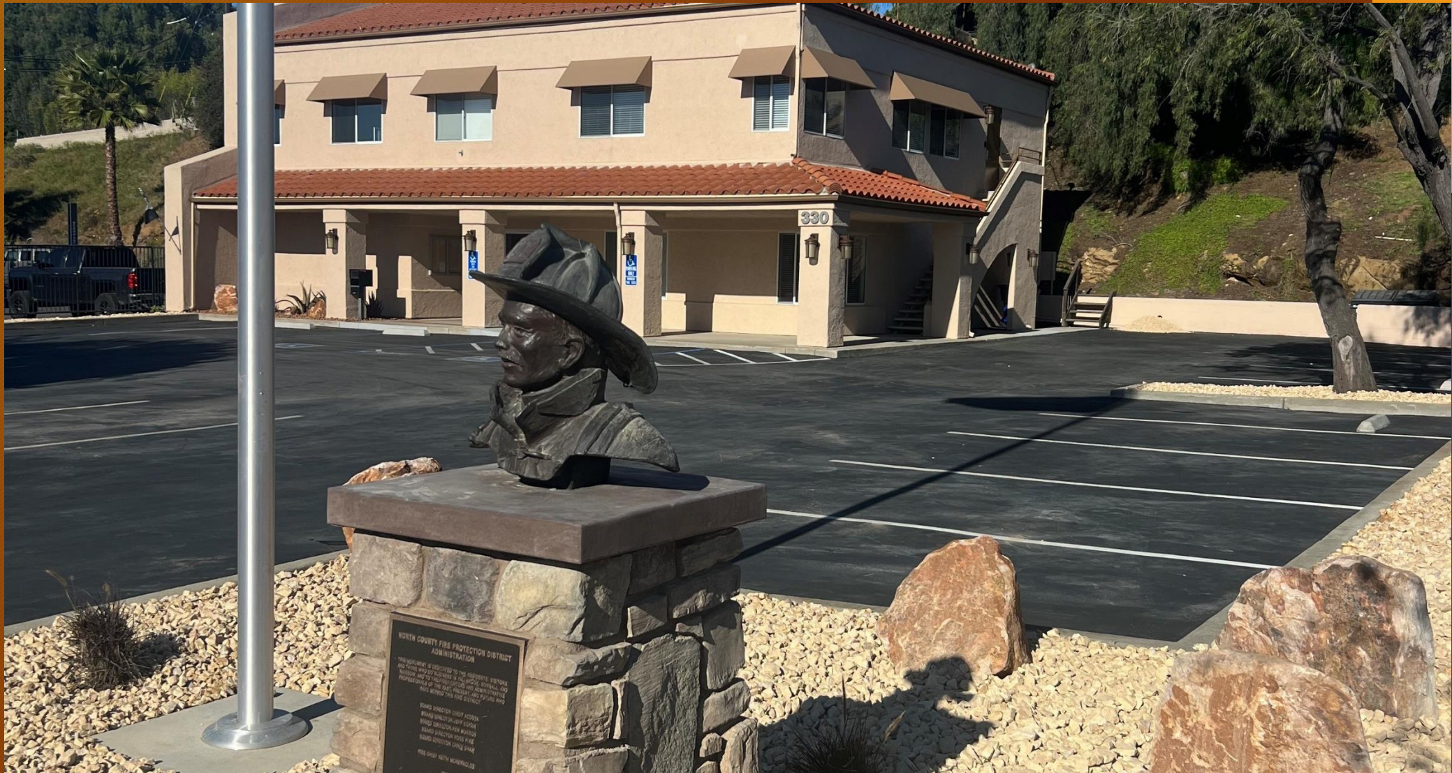
Fire Administration Renovation, 2024
